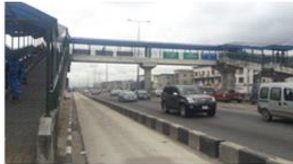
Figure 4.1b: Pedestrian Bridge at Fadeyi Bus Stop
