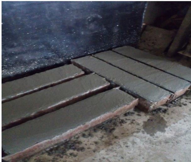
Plate 3: Casting of the Beams
