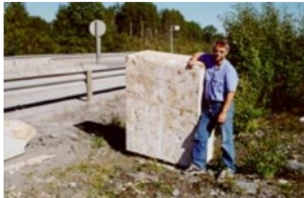
Figure 3: Excavation of a 24 years old EPS block used for embankment at Flom bridge in Oslo Norway. (Tomasz et al. , 2019)
