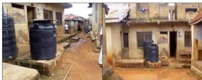
Figure 5. Storage tanks used for public water supply
