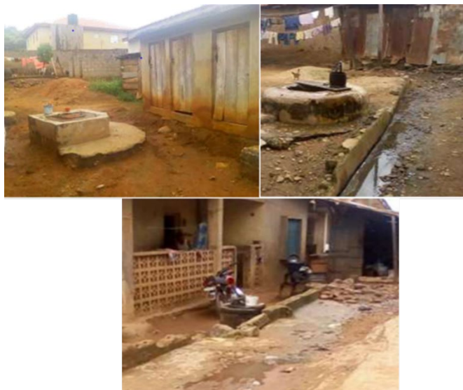
Figure 4. Unsanitary condition of hand-dug wells in Ado-Ekiti
